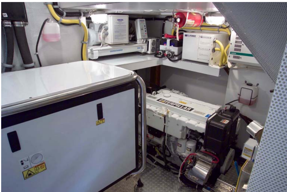
THE ENGINE ROOM IS NEATLY DETAILED WITH EXCELLENT ACCESS TO ALL MACHINERY.
